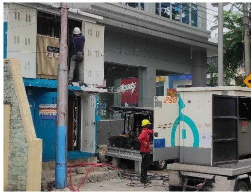
Figure 5. Utilization of Mobile Transformer Units On Transformer Maintenance
